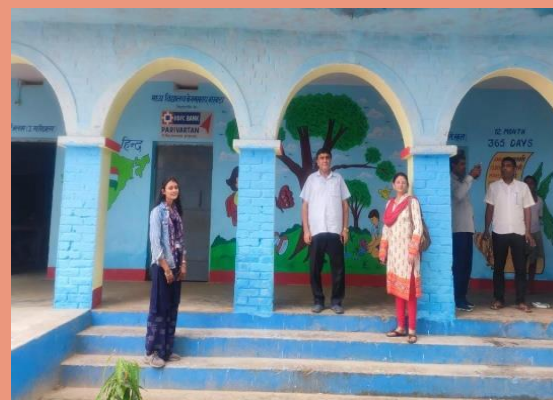
Renovated Middle School, Begumsarai, Bachhwara
